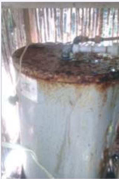
Leaking hot water system
